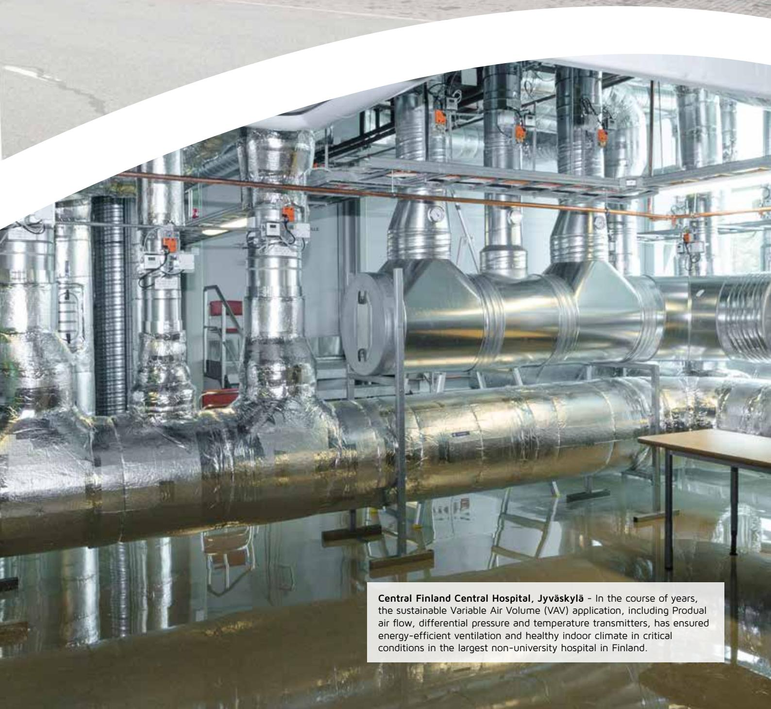
**Central Finland Central Hospital, Jyväskylä** - In the course of years, the sustainable Variable Air Volume (VAV) application, including Produal air flow, differential pressure and temperature transmitters, has ensured energy-efficient ventilation and healthy indoor climate in critical conditions in the largest non-university hospital in Finland.
